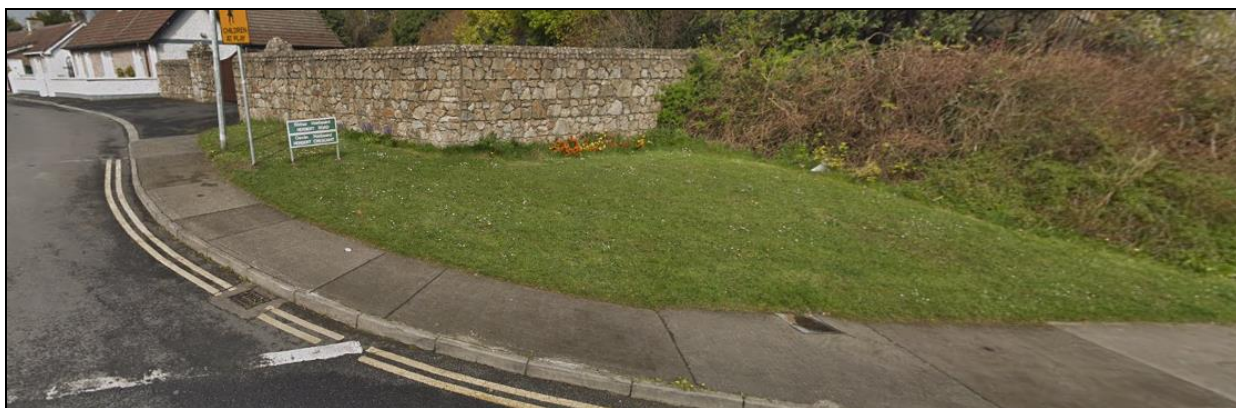
Plate 6: Location of R5-TP05 and R5-RC03 facing NW.
